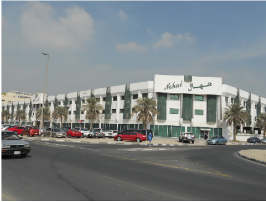
G+3F+R Building at Al Qusais, Dubai
