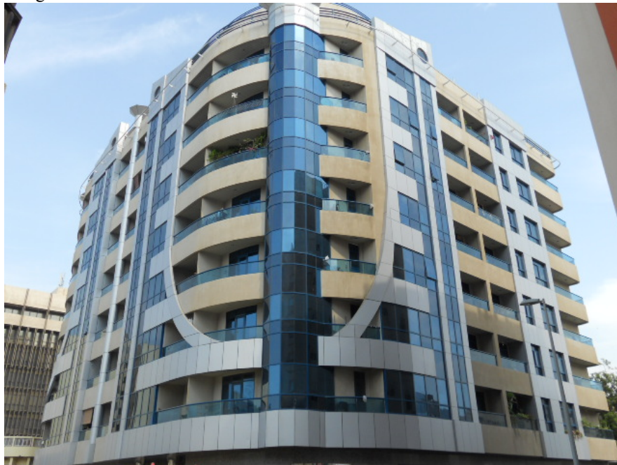
G+7F+R Building at Bur Dubai
