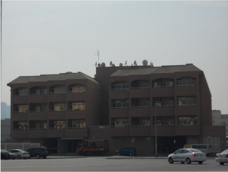
G+4F+R Building at Bur Dubai
