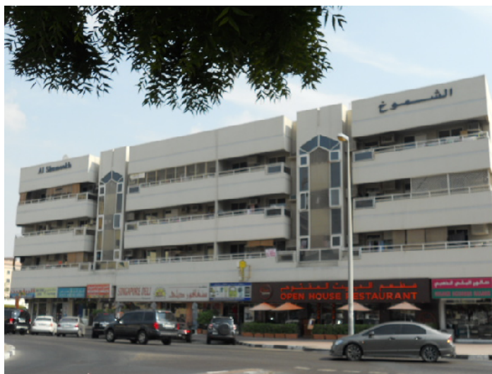
G+3F+R building at Al Karama, Dubai
