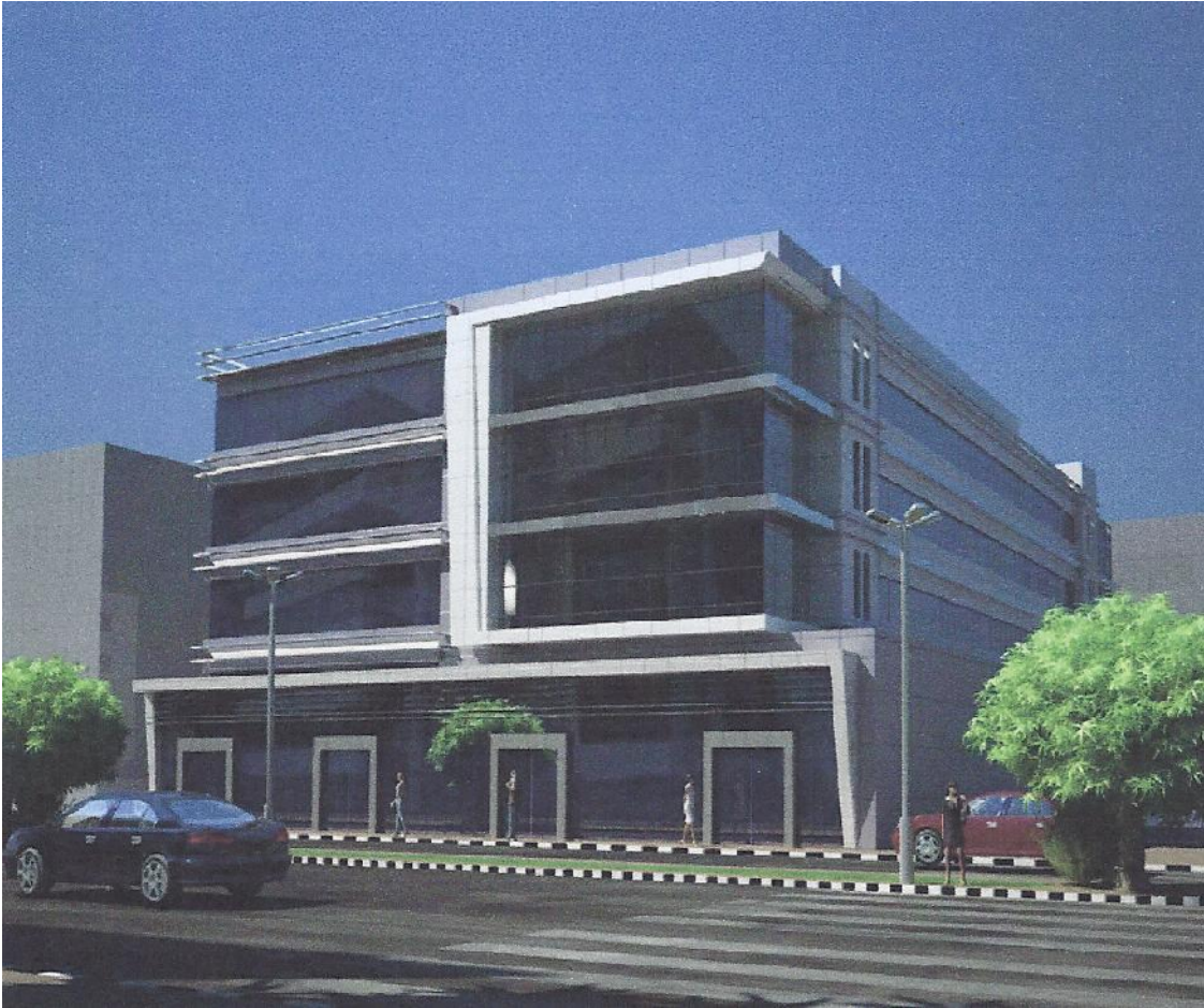
Umm Hurair hospital building
