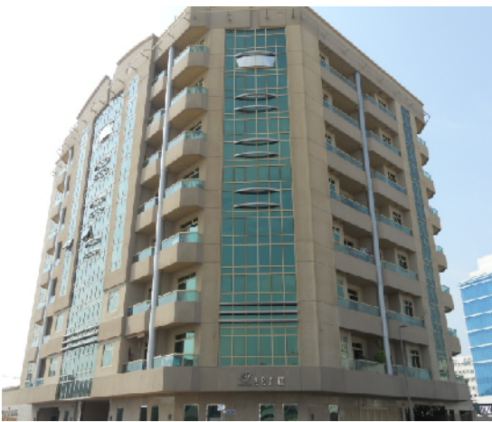
G+7F+R Building at Bur Dubai
